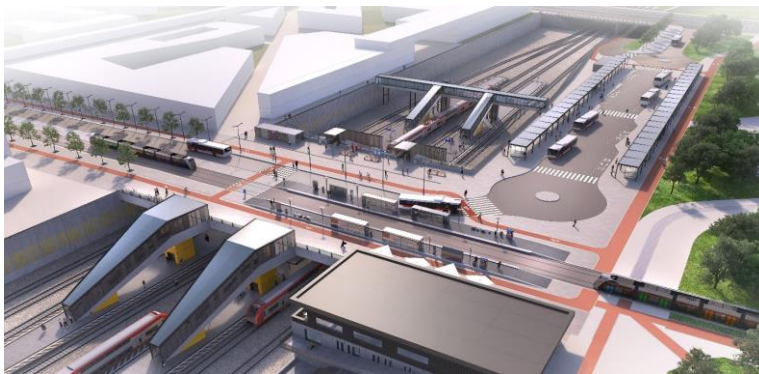
Future Howald train station and multimodal hub (2024)
