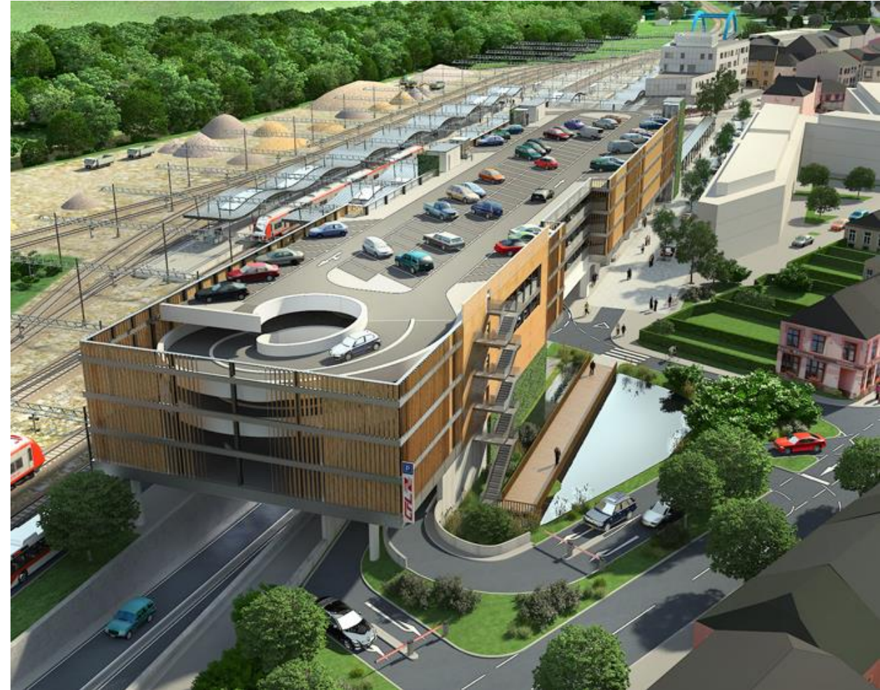
More than 400 parking spaces will be available at P&R Ettelbrück by 2023 (source CFL)
