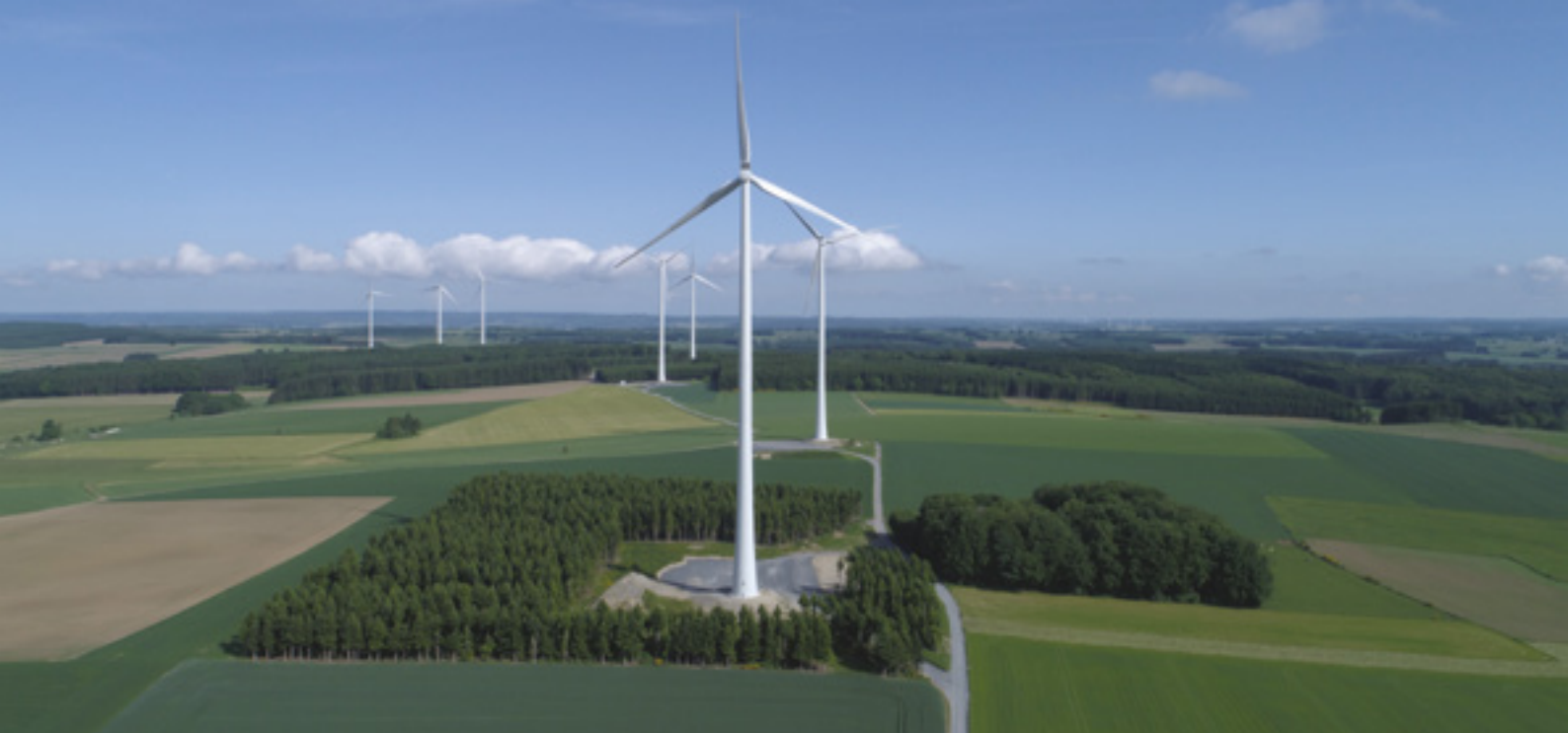
/ Wind farm – Wincrange /
